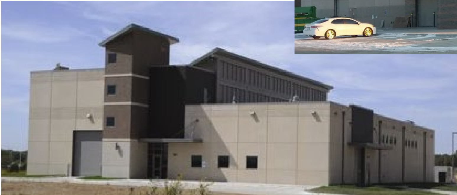
County Adult Detention Thermal Facility (2012)
