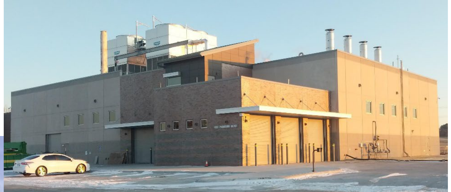
Nebraska State Penitentiary Thermal Facility (2019)
